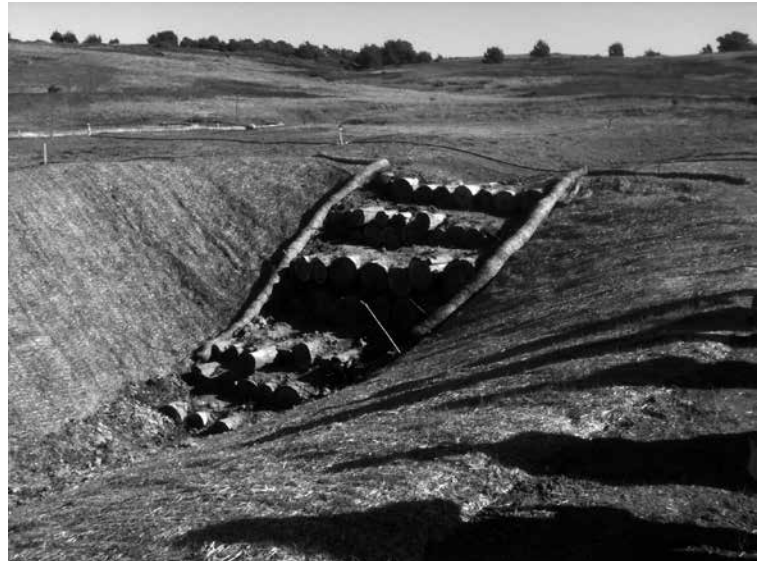
A log headcut repair site near Cambria, CA.
