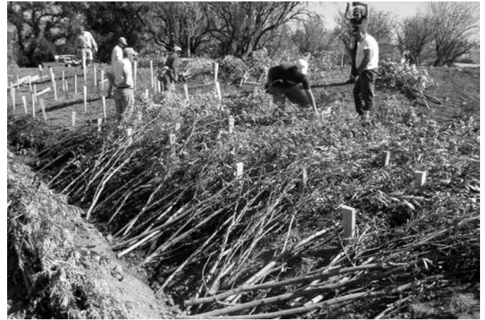
Volunteers install a brush mattress.
