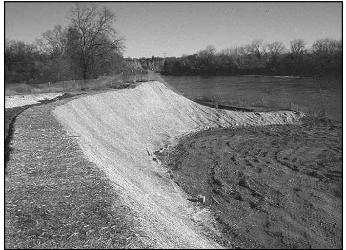
Erosion Control Blankets installed at a construction site.
